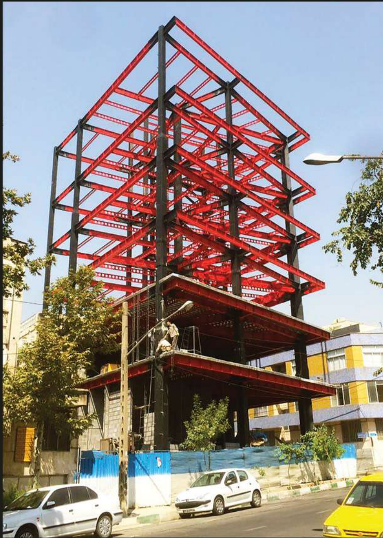
Haft-e-tir Project (Noori esfandiari alley) Bolts installation WUF-W,BFP 250tons
