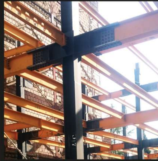
Manzarie project Bolts installation WUF-W,BFP tons 270
