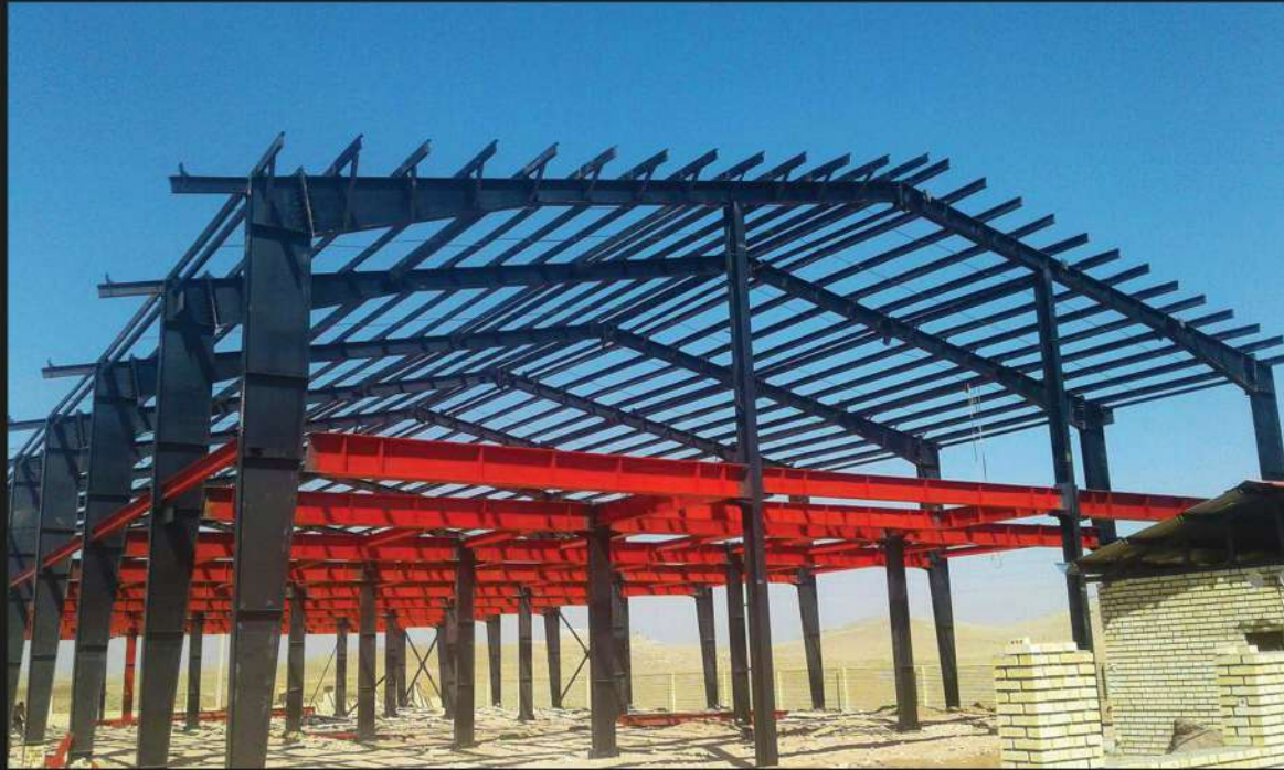
Artiman factory Project Welding connection tons 100
