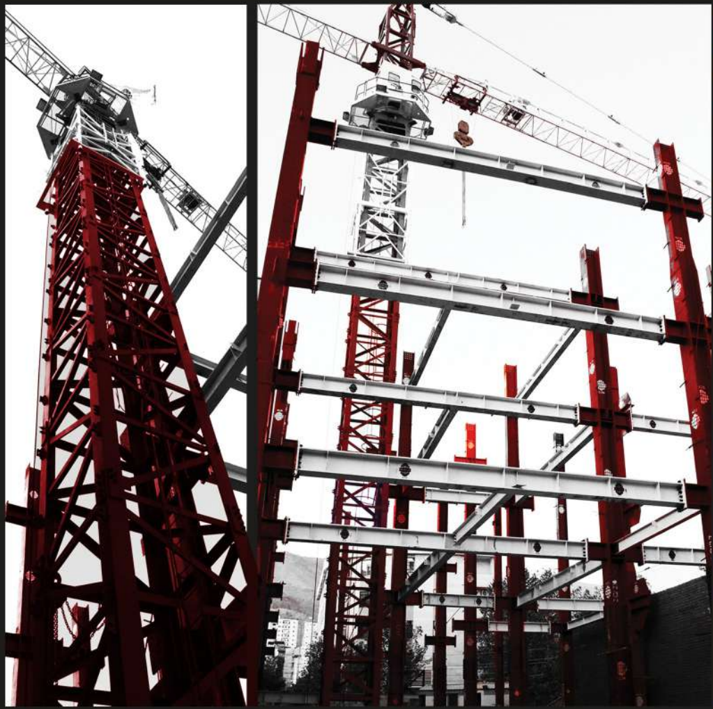
Andarzgoo Project (South Salimi) Bolts installation BSEEP 800tons
