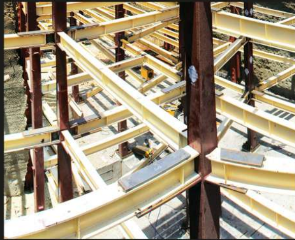
Jannat Abad project Welding connection WFP 800tons
