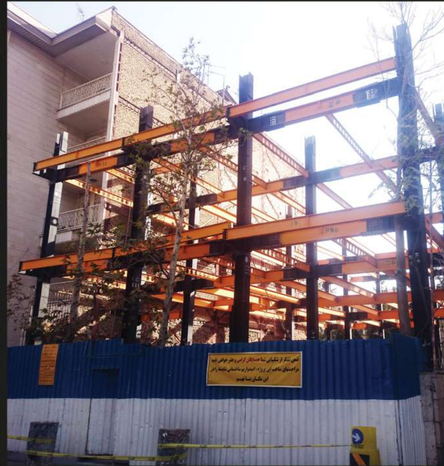
Manzarie project Bolts installation WUF-W,BFP tons 270
