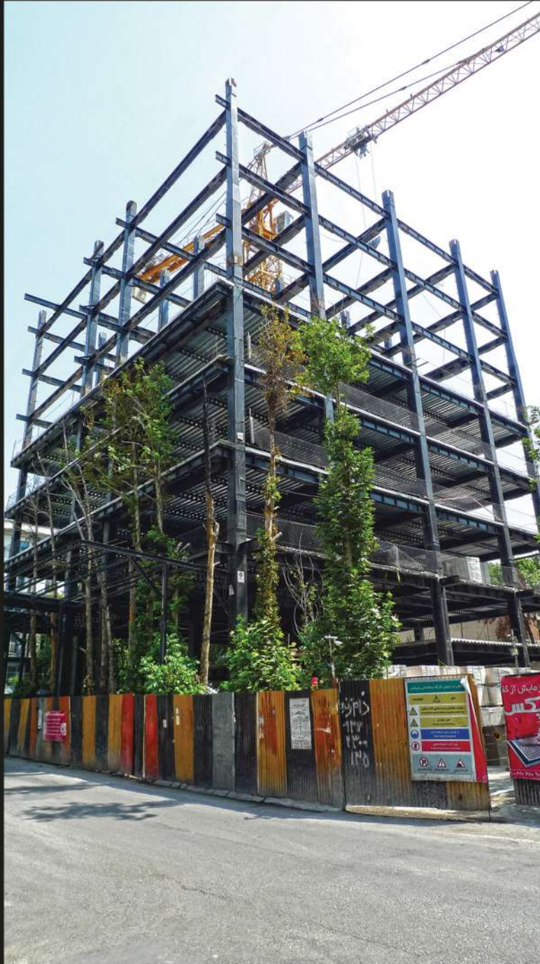
Elahie project (mixed-use building) Welding connection WUF-W,WFP tons 1800
