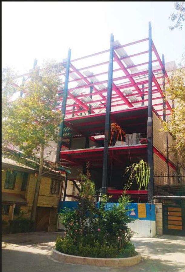
Farmanieh project (Saadi) Welding connection WFP 270tons
