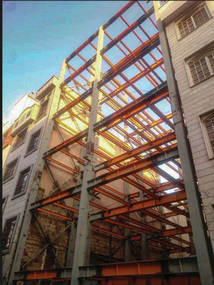
Fatemi Project Bolts installations WUF-W,WFP 120tons
