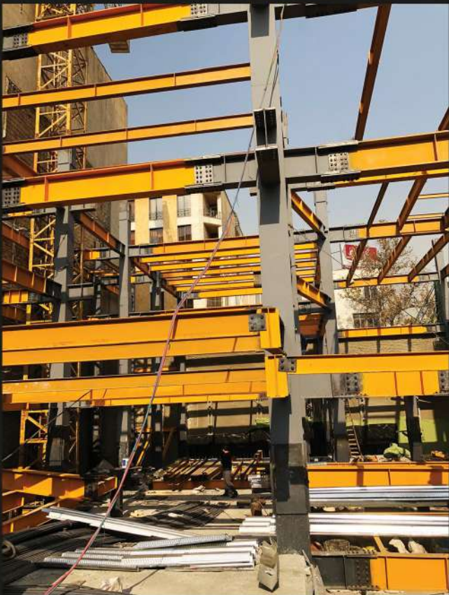
▶ Pasdaran rabi project (Across from Golestan 7th) Bolts installation WUF-W,BFP 900tons
