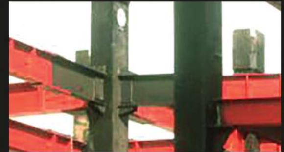
Qeytarie project Welding connection WFP 300tons
