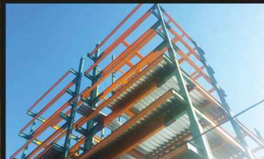
Heravi project Commercial and residential Welding connection WUF-W,WFP 300tons
