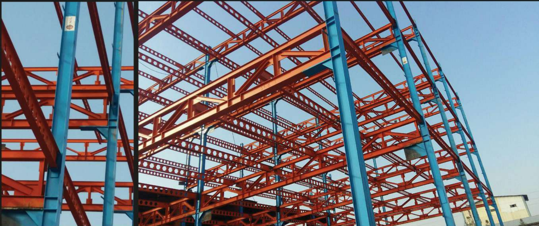
Shoepa shoe factory Project Welding connection tons 120
