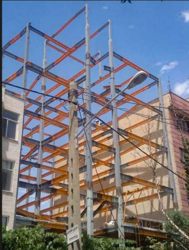
◀ Jolfa Project Bolts installation WUF-W,WFP 150tons
