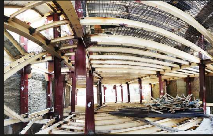
Vozara project Welding connection WFP 1000tons ◀
