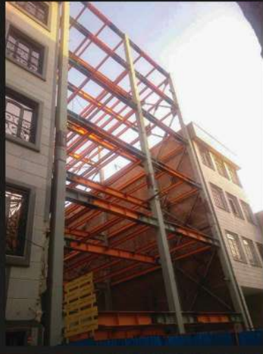
Fatemi Project Bolts installations WUF-W,WFP 120tons
